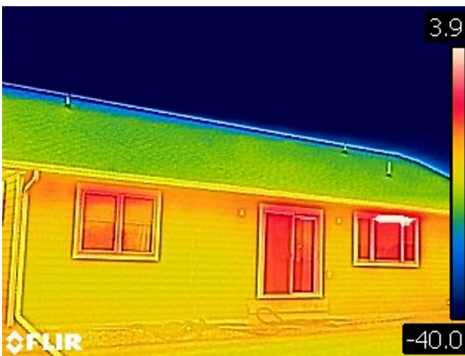
IMAGE 1.7: MINNESOTA SIP HOUSE (THERMAL)
