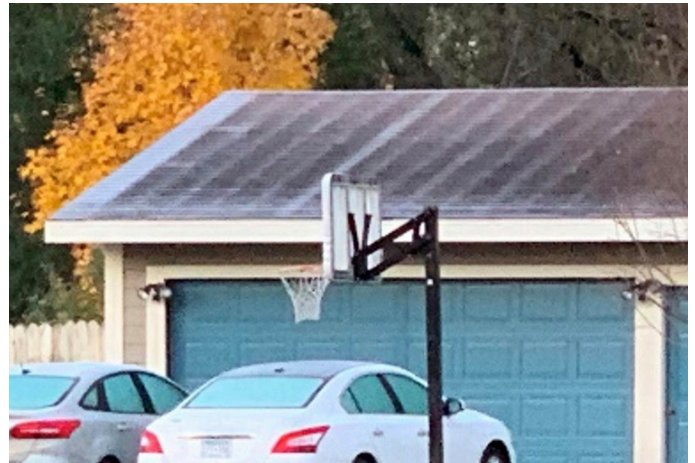
IMAGE 1.4: TRADITIONAL GARAGE ROOF
