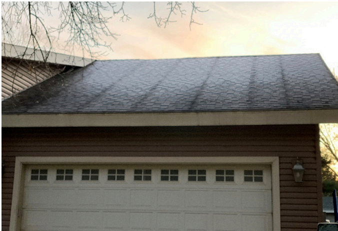
IMAGE 1.3: SIP GARAGE ROOF
