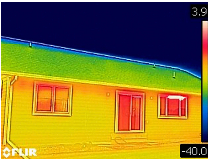
IMAGE 1.7: MINNESOTA SIP HOUSE (THERMAL)
