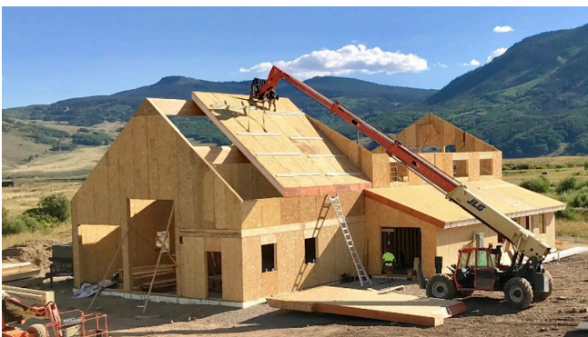
IMAGE 7.31B ROOF SIPs WITH TOE BOARDS
