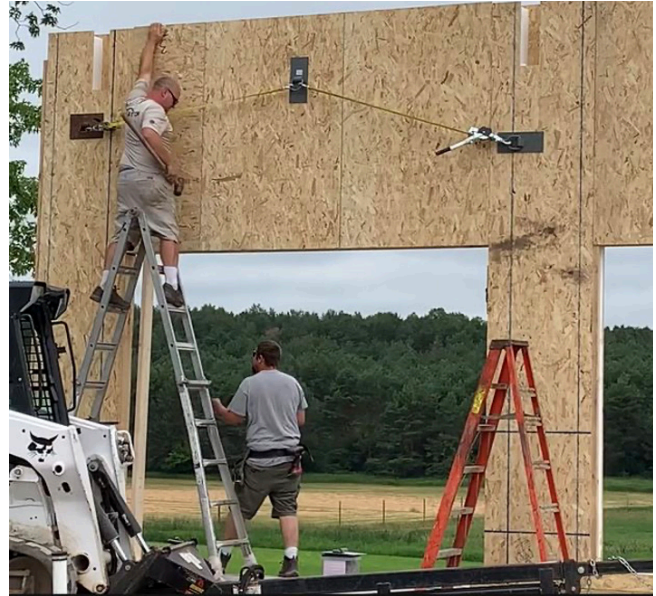
IMAGE 7.22B USING RATCHET STRAPS TO PULL SIPs TOGETHER
