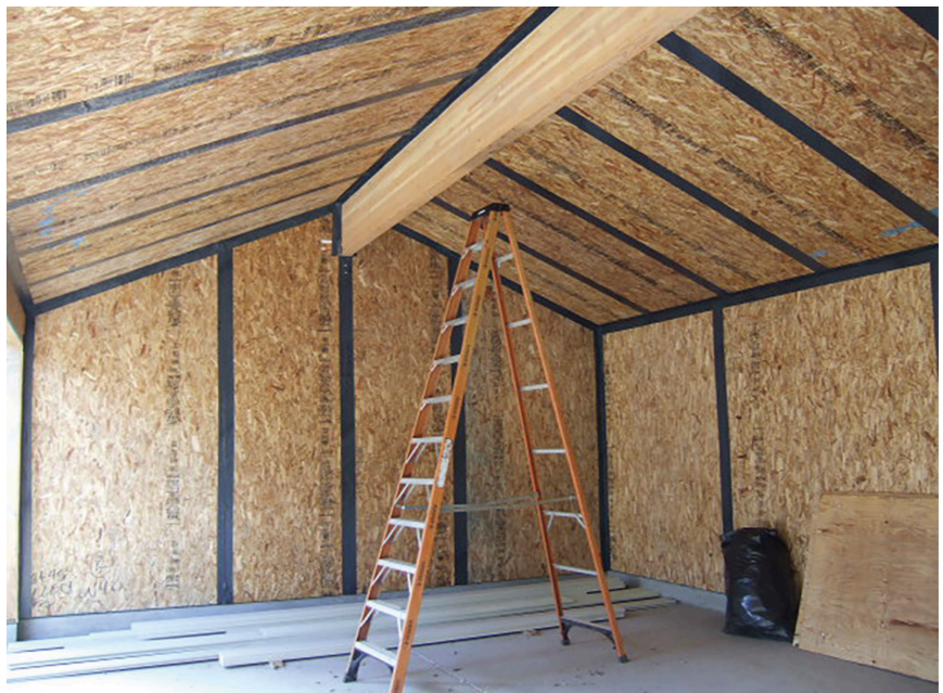
IMAGE 7.38 SIP TAPE APPLIED TO INTERIOR SIP ROOF AND SIP WALL JOINTS
