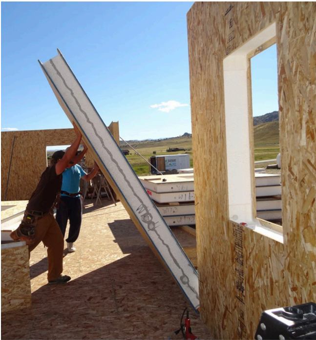
IMAGE 7.4 SIP WALL SEALANT APPLICATION
