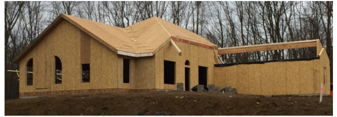
IMAGE 7.31E ROOF SIPs WITH TOE BOARDS
