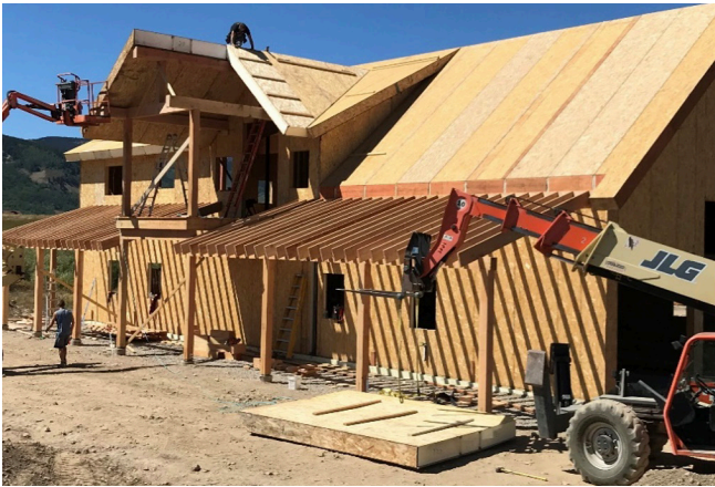
IMAGE 7.31A ROOF SIPs WITH TOE BOARDS
