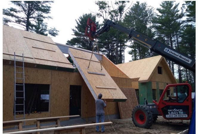
IMAGE 7.31C ROOF SIPs WITH TOE BOARDS
