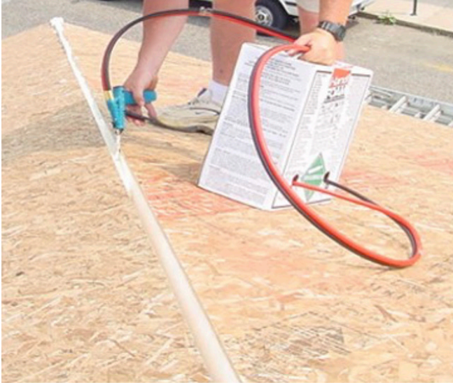
IMAGE 7.2 EXPANDING FOAM INSULATION AT SIP ROOF RIDGE JOINT
