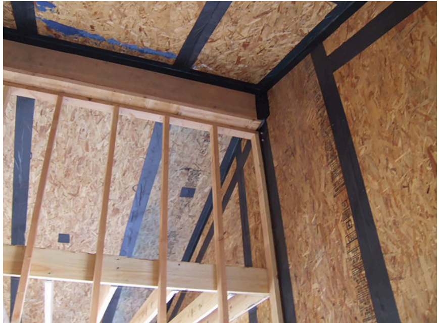
IMAGE 7.38 SIP TAPE APPLIED TO INTERIOR SIP ROOF AND SIP WALL JOINTS
