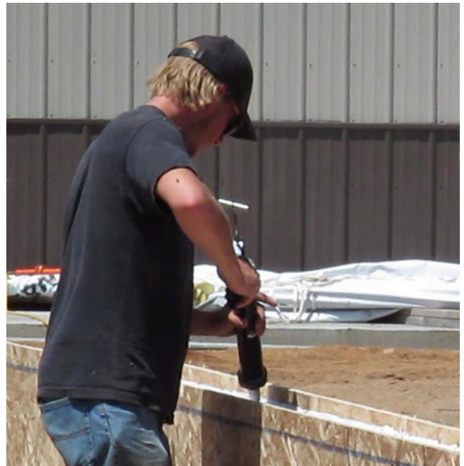
IMAGE 7.5 SIP WALL SEALANT WITH MANUAL APPLICATOR
