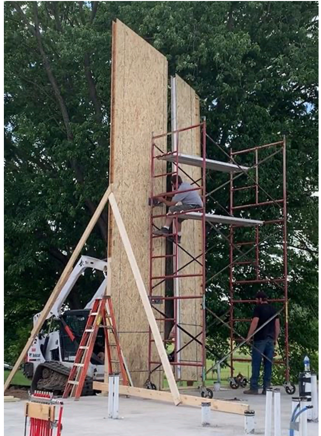
IMAGE 7.28 EXTERIOR SIP WALL BRACING FROM THE EXTERIOR OF THE BUILDING
