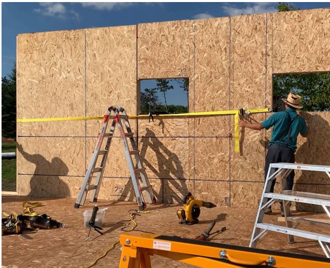
IMAGE 7.22A USING RATCHET STRAPS TO PULL SIPs TOGETHER
