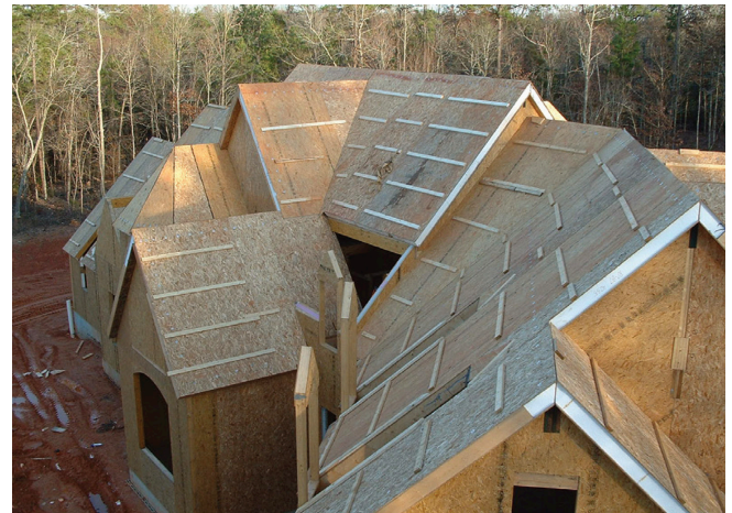
IMAGE 7.31E ROOF SIPs WITH TOE BOARDS
