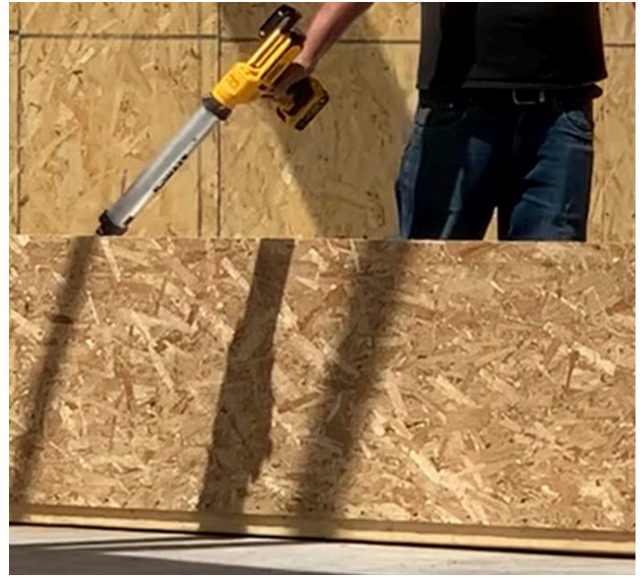
IMAGE 7.3 AUTOMATED SEALANT APPLICATOR
